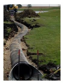
Figure 17. Drainage pipe installation.
