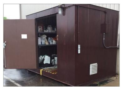
Figure 46. Proper chemical storage.
