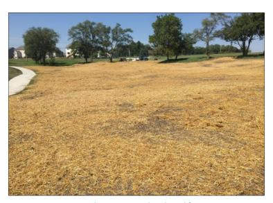
Figure 2. Straw is used to protect soil and seed from water erosion.
