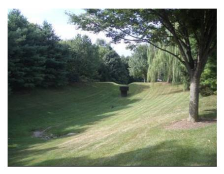
Figure 8. Use dry detention basins/catchments to buffer flooding and excessive runoff that may contain sediment. Photo credit: Kraig Binder.
