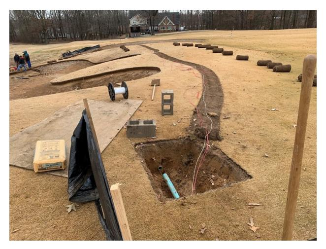
Figure 4. Irrigation systems should be properly designed and installed to improve water use efficiency. Photo credit: Shannon Watson.
