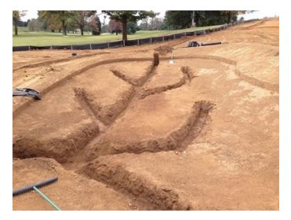
Figure 2. When constructing drainage systems, pay close attention to engineering details such as subsoil preparation, the placement of gravel, slopes, and backfilling. Photo Credit: John Ballard, CGCS.
