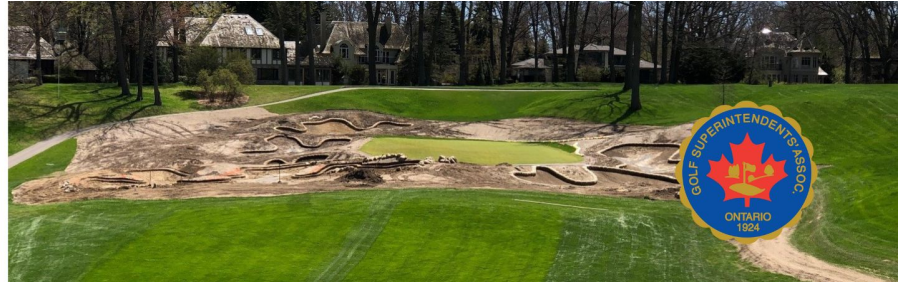
St. George's bunker construction. OGSA image. ONCourse, August 2019, pg. 22.
