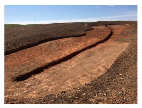
Figure 4. Bunker drainage.
