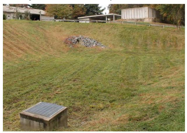
Figure 13. Retention ponds temporarily hold water from storm events.
