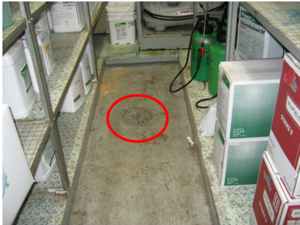
Pesticide stored in a room with an open drain.
