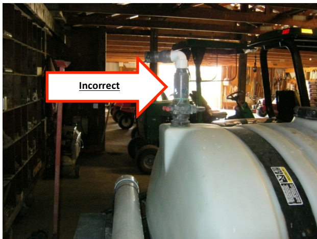
No physical separation in air gap
