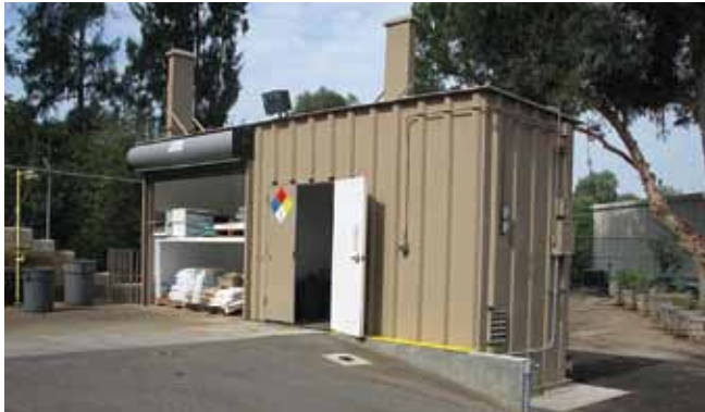
An example of a fertilizer and pesticide storage facility.
