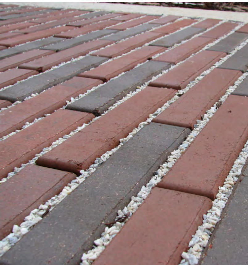
Figure 4 and 4.1 Maximize the use of pervious pavements. Grass is usually only suitable in between pavers when a soil is engineered to retain nutrients and appropriate moisture. The use of “grass-crete” is not recommended for high-traffic areas without irrigation and proper maintenance.
