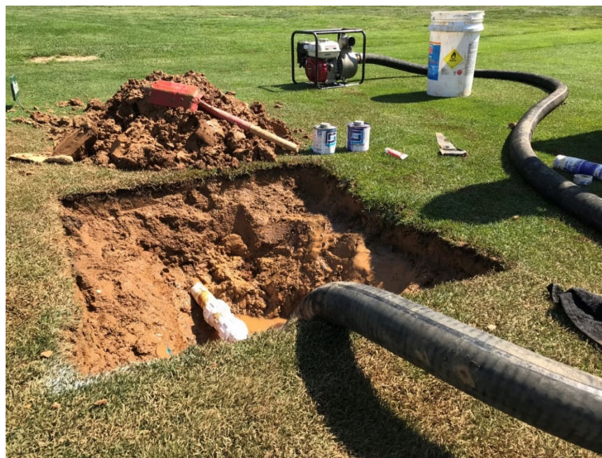
Figure 6. Irrigation system maintenance.
